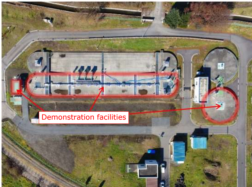
Photo 1. Full view of demonstration facilities
