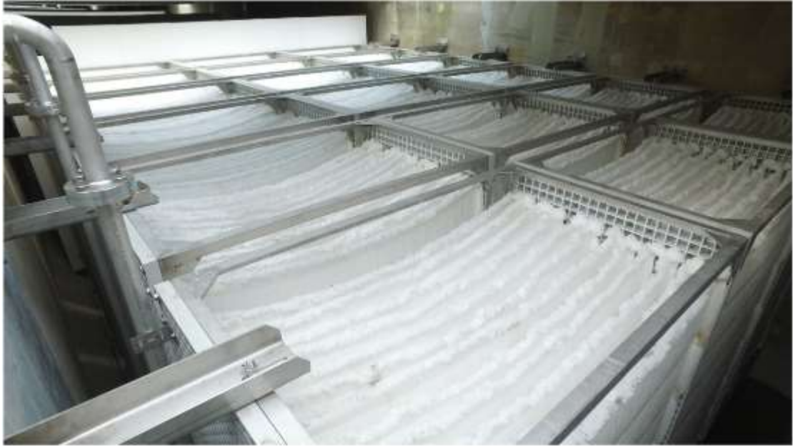
Photo 3. Setting condition of special fiber carrier (Inside of reactor)
