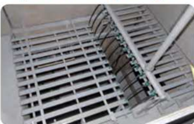
Low pressure loss membrane diffuser
