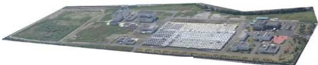
Ban-nan WWTP overview
