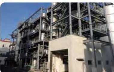
Next generation type incineration system
