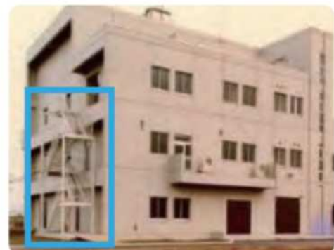
Example of tsunami control measures (Installed outdoor stairs)
