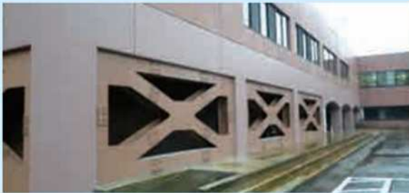
Aseismic construction by concrete braces reinforcement
