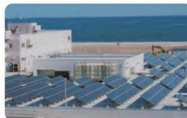
Solar power generation
