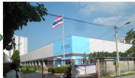
Achievement of support: beautifully renovated Siracha WWTP, Thailand
