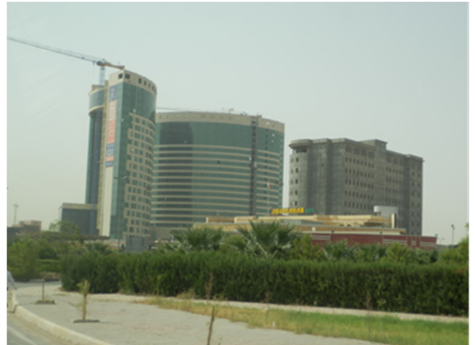
Photo 6: Still-under-construction tower building
