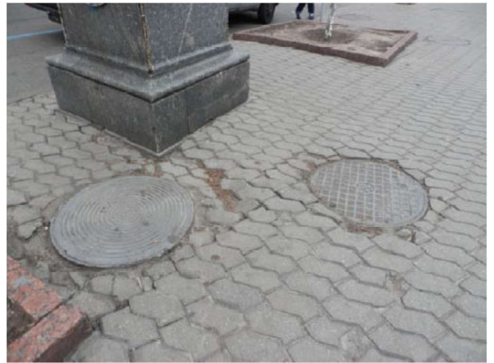
Photo 2: Two kinds of a manhole cover: wastewater and rainwater
