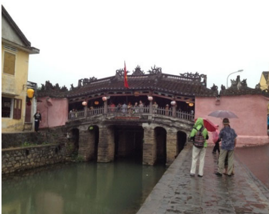
Photo1: Japanese Bridge in Hoi An City
