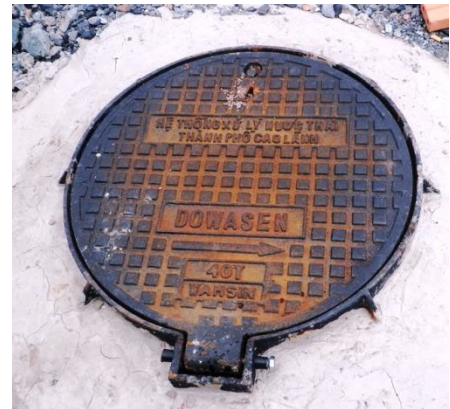
A manhole in Dong Thap Province
