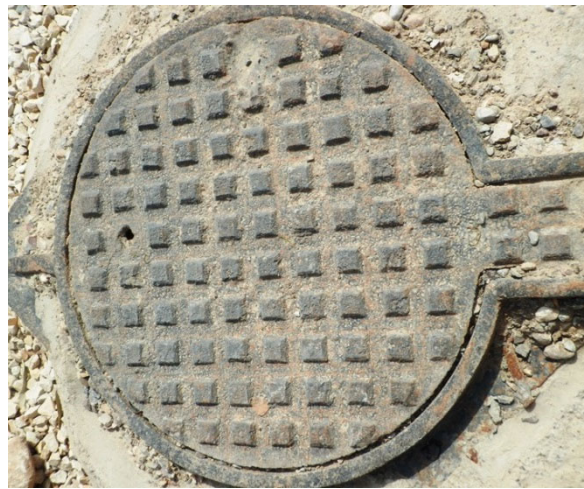
A manhole of Citadel of Erbil
