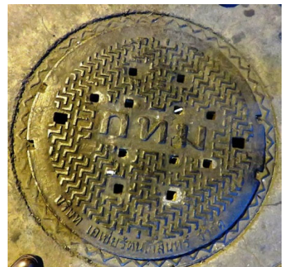
A manhole in Bangkok,
