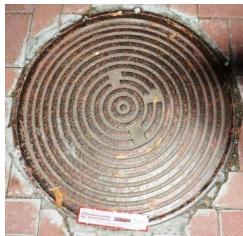
A manhole of Kyiv #2
