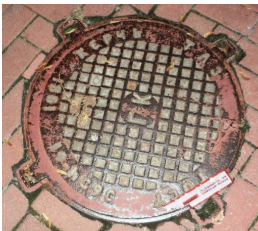
A manhole of Kyiv #1
