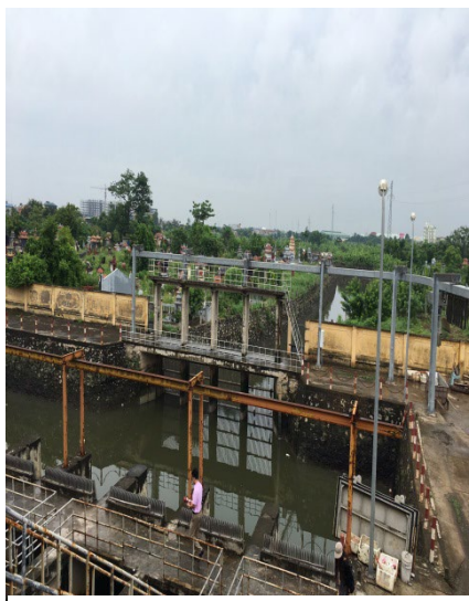
Photo 2: Channel to pump station
