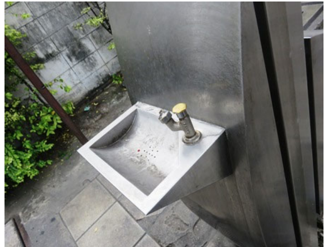
Water fountain on the sidewalk in Bangkok
