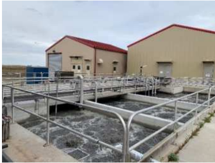
Photo 1. Leading-edge sewerage system (MBBR)
