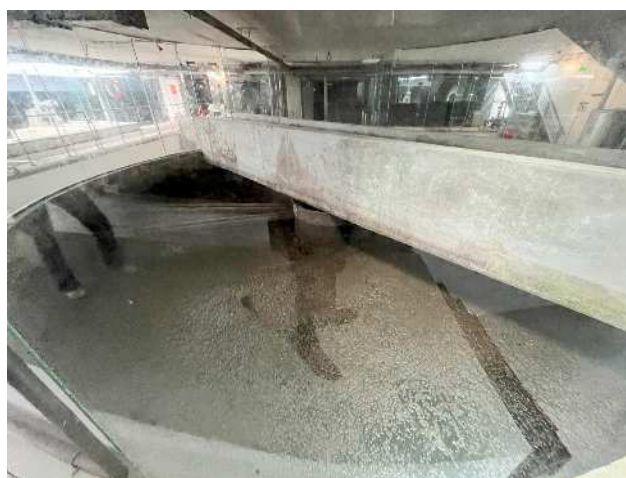
Glass-fronted gravity thickening tank
