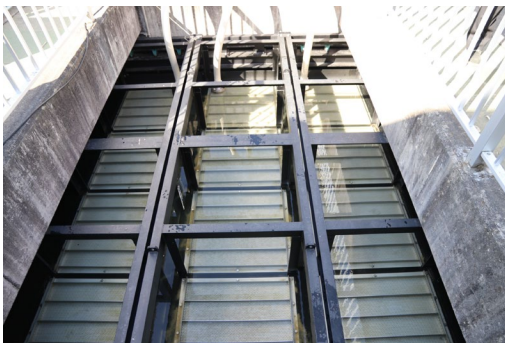
The upper part of filtration area
