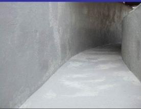
The thickness of sulfuric acid-resistant mortar was set to 10mm, based on the prediction of deterioration. The thickness of cross-sectional restoration material (10mm) plus sulfuric acid-resistant mortar (10mm) or sulfuric acid-resistant mortar (20mm) was used, depending on the performance of each material.
