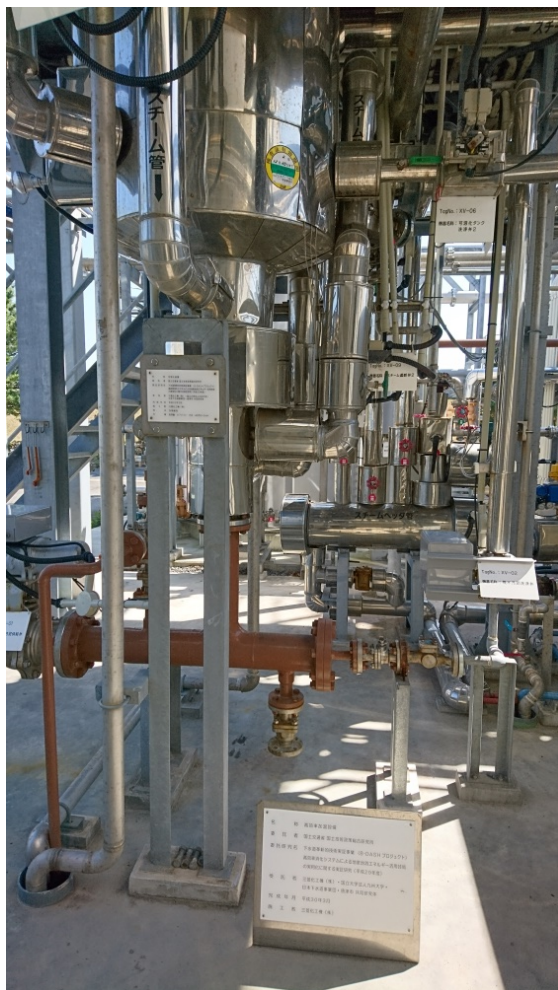
Solubilization device (highly efficient heating system)
